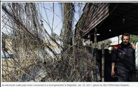
An electrician works past wires connected to a local generator in Baghdad, Jan. 23, 2011. (photo by Reuters/Donna Strassman)
